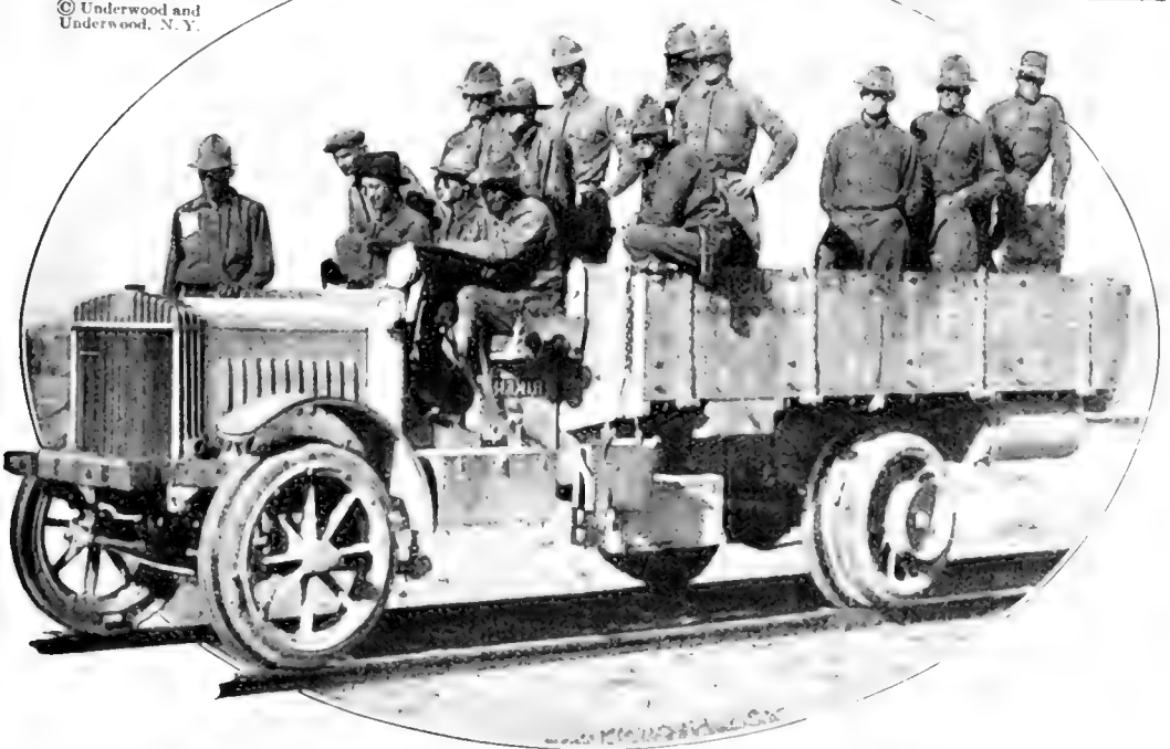
At the end of a six days' march southward into Mexico. With the limited forces and inadequate equipment at their disposal, the United States troops have acquitted themselves very creditably. The truck shown is equipped with flanged steel rims fitted over the wheels. It can run on the railroad tracks, and with but slight alterations can again take to the roads. Several of these versatile vehicles were recently forwarded to our army at Columbus, New Mexico
